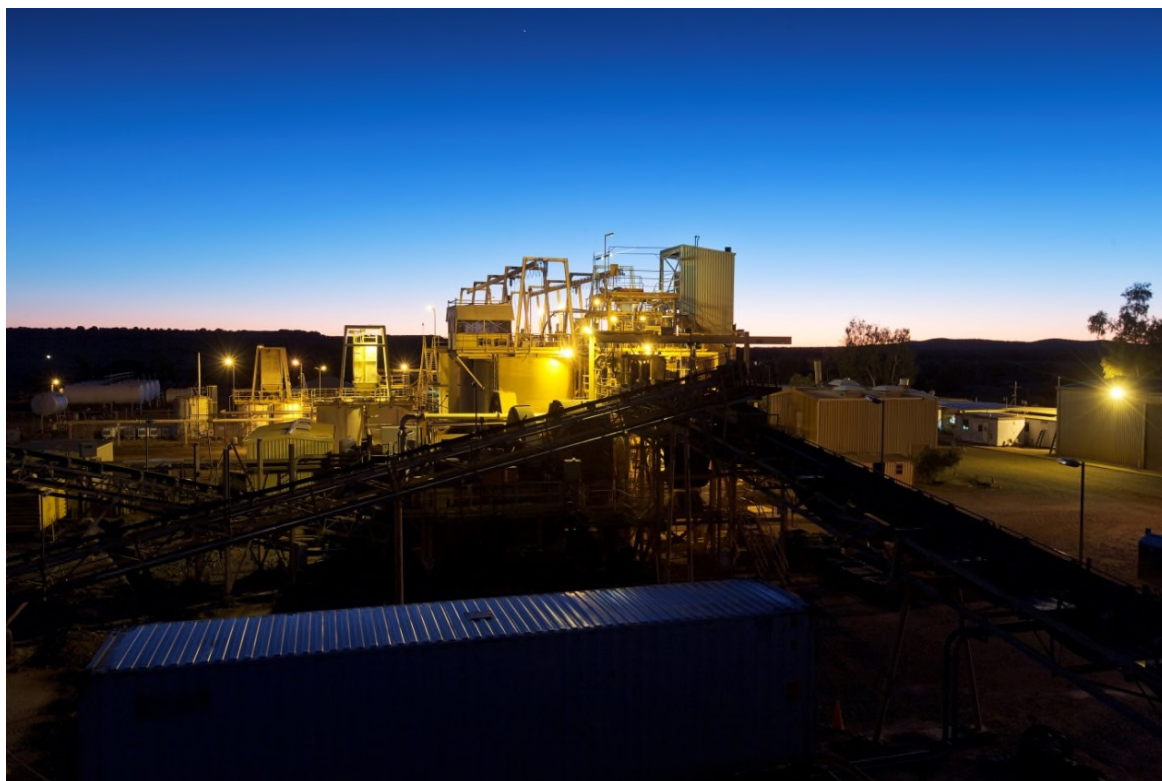
1Mtpa Grosvenor gold treatment plant
