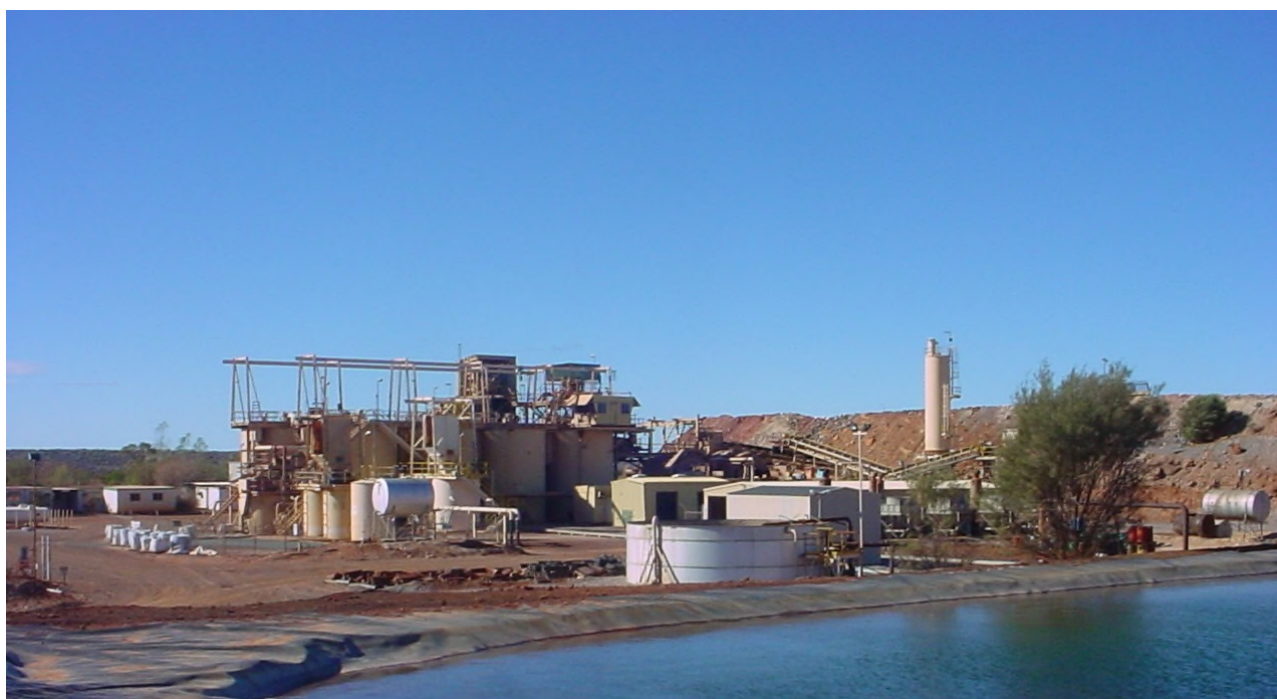
Figure 1: Grosvenor CIL gold processing plant
